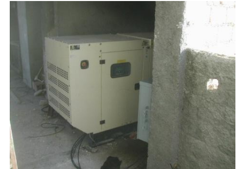
Generator finally in place and hooked up.
