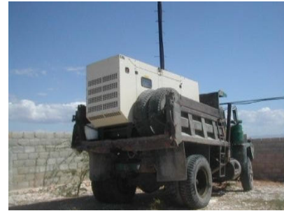
Generator just prior to unloading.
