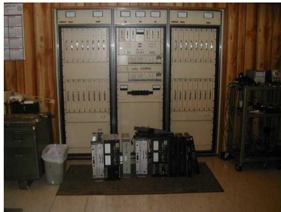
WRTV Transmitter and other analog equipment (on mat) prior to disassembly.
