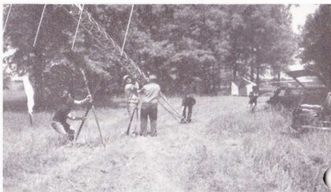
Lowering of the antenna — Mike Lennen, KDØEV; Jim, NØAIH; Frank, WDØESL; Dave, NØCLW; Greg, NØBTN; and not in view, Mitch, NØAZF.
