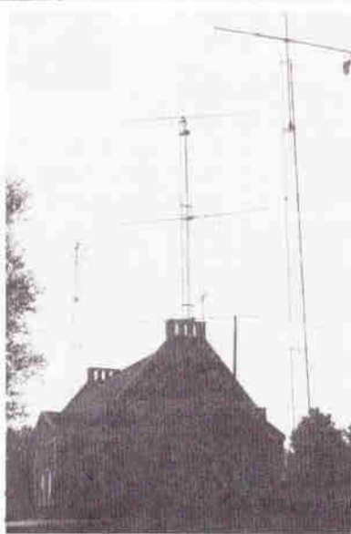
W1AW Building - showing some of the antennas
